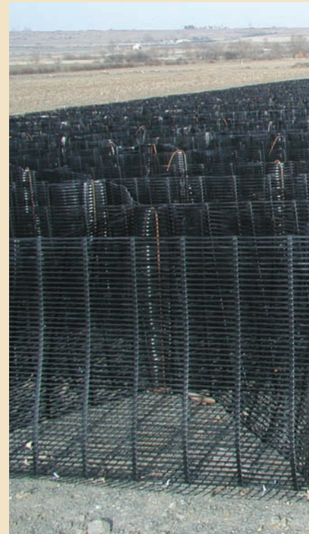
2. Rapid site assembly of Tensartech Geocell Mattress System
