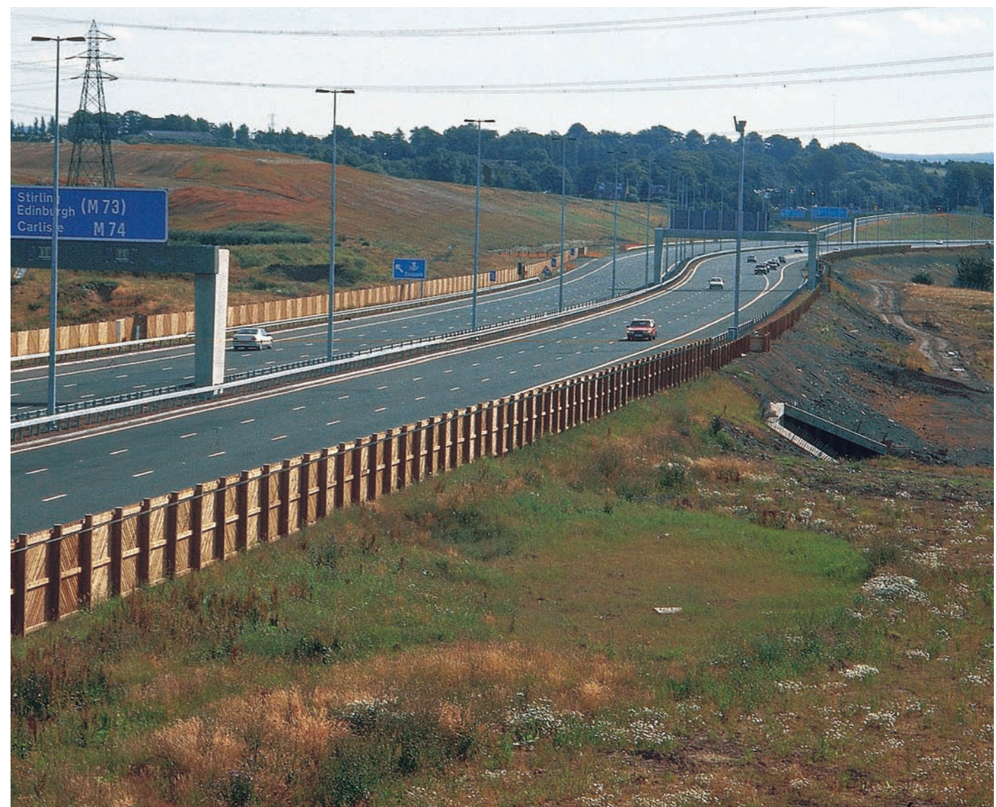
The TensarTech Geocell Mattress System provides stiff basal support in the control of differential settlement on the M74, UK.
